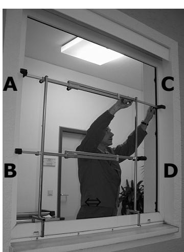
Once the opposing extension brackets **C** and **D** have been pulled out to the maximum width of the window, the safety railing is securely locked into place on the window frame.
